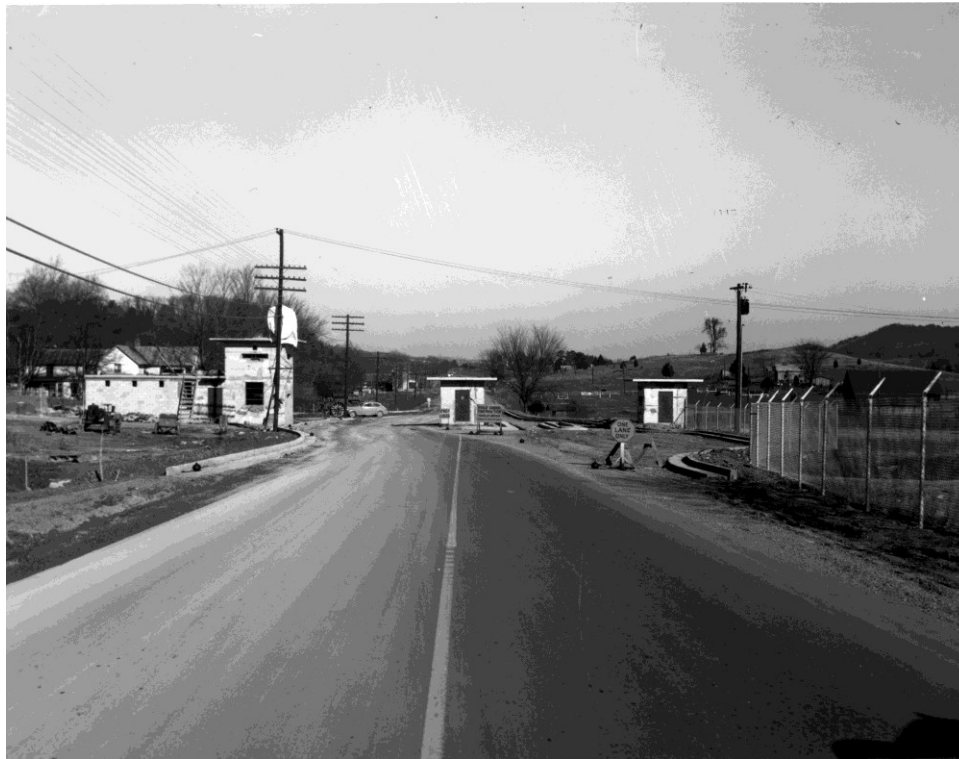
Construction of the "Checking Station" on the Oak Ridge Turnpike (Photo by Ed Westcott)
