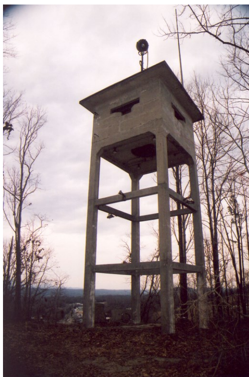
Close up view of the Observation Tower atop Pine Ridge
