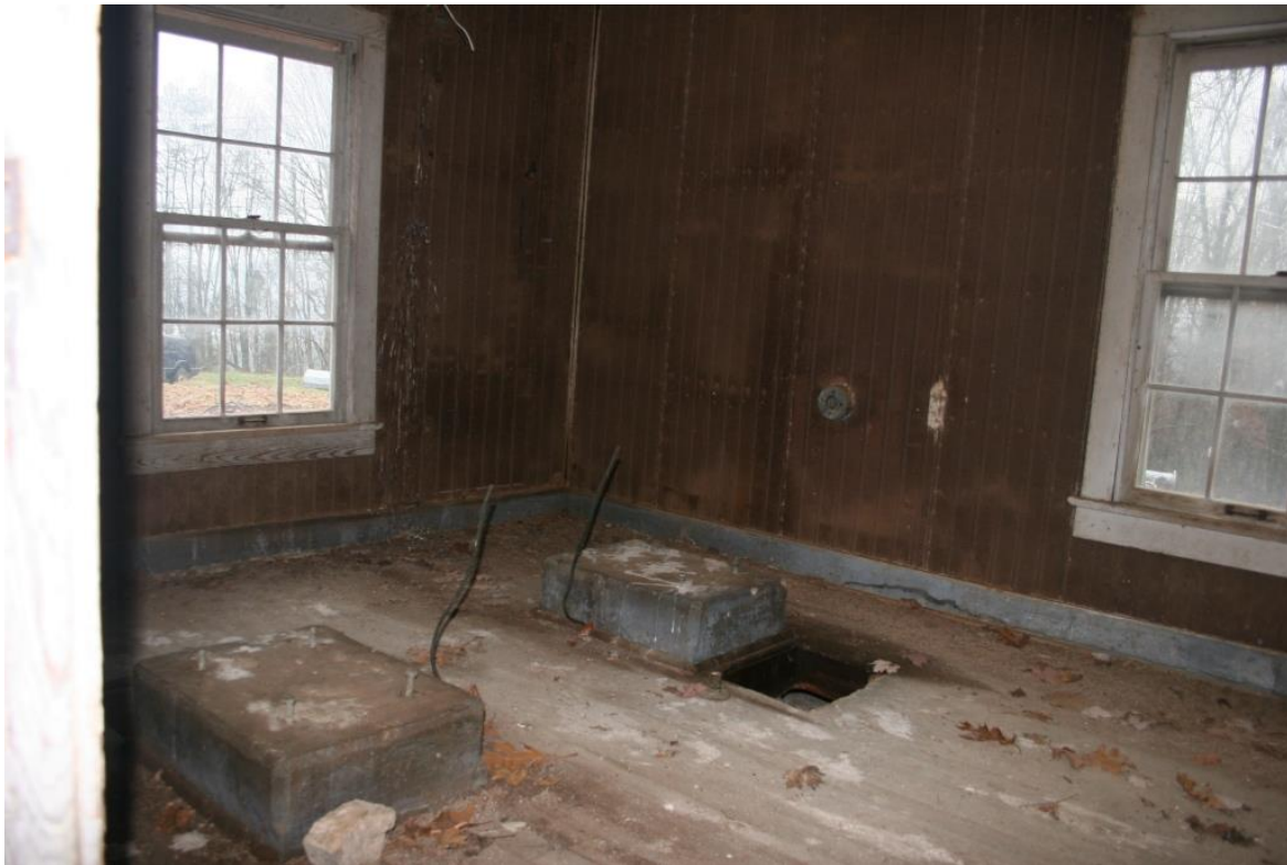
Interior of Beacon House showing concrete footers on which the generator sat that powered the airway light
